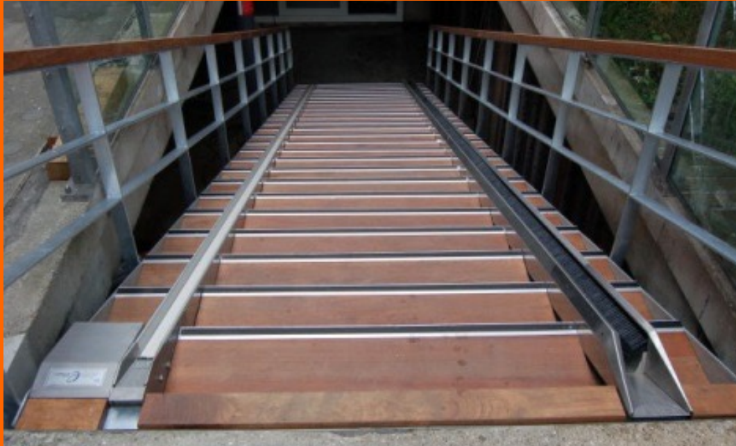
Location: Amsterdam, Holland Installed : April 2014 Length: 33' [10 m] Outdoor
