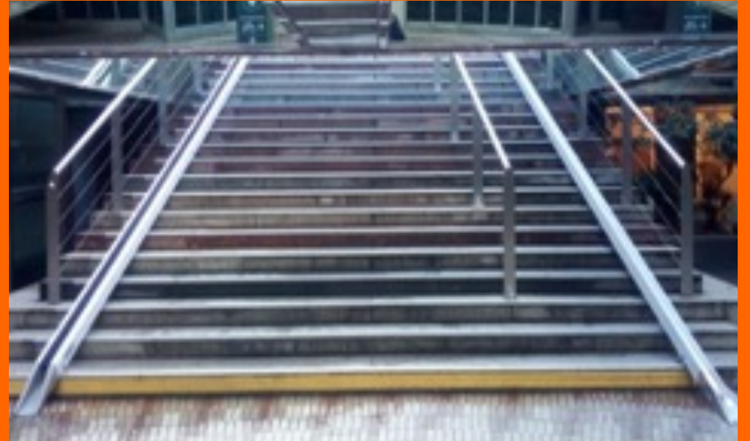
Location: Paris, France Installed: September 2019 Length: 46' [14 m] Outdoor
